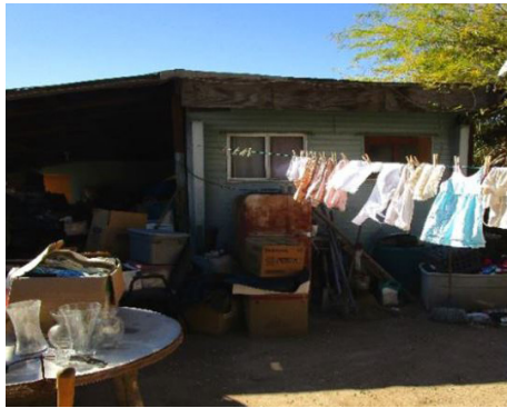
City of San Luis Home Rehab Project (Before)
