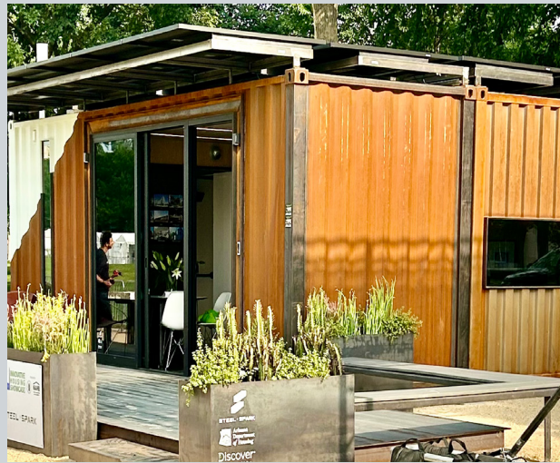
In FY 2023, ADOH funded the design and construction of the SparkBox; an innovative, solar-powered, quick-occupancy housing solution using repurposed shipping containers
